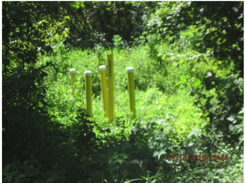
Piezometer at site 11.
