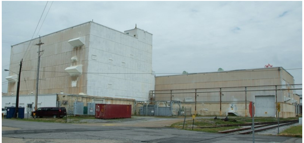
C410/420 building before demolition.
