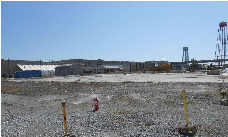
C410/420 slab after demolition.
